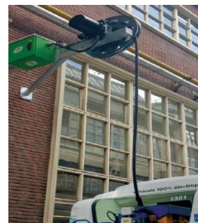
Figure 13 - Example of wall mounted cable reel
