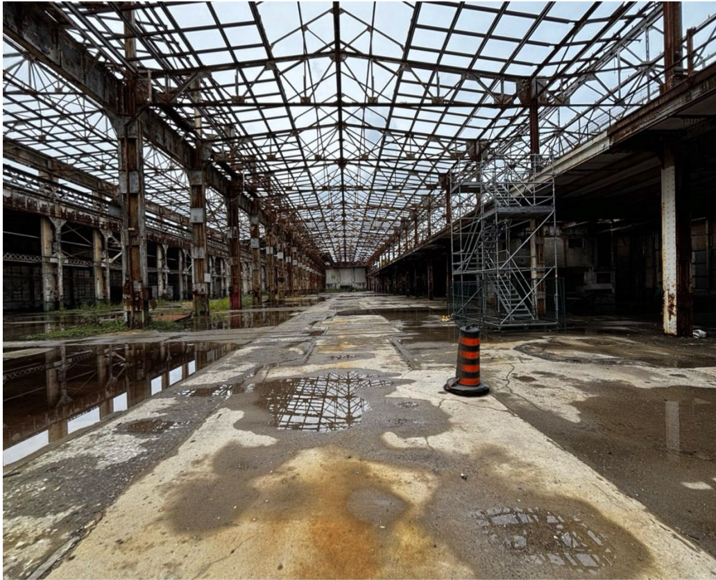
INTERIOR VIEW LOOKING WEST
