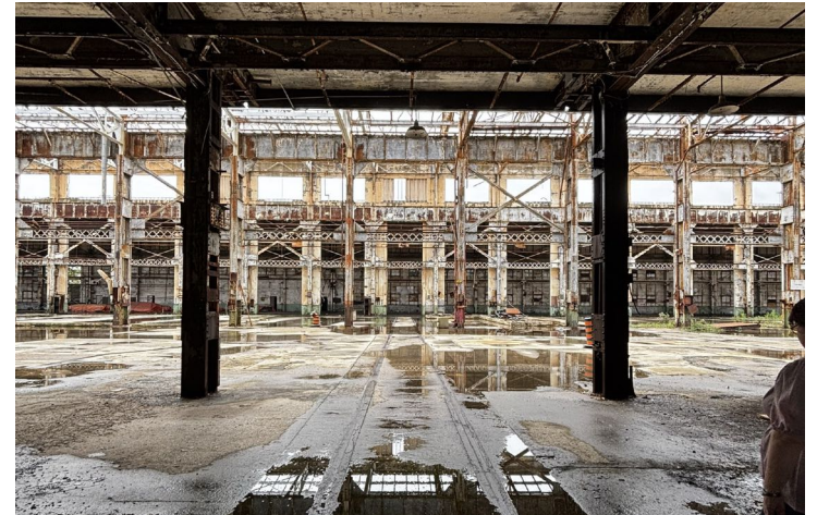
INTERIOR VIEW OF MEZZANINE FROM UNDERNEATH
