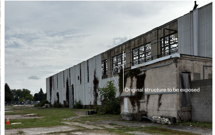
EXTERIOR VIEW OF FACADE LOOKING SOUTHWEST
