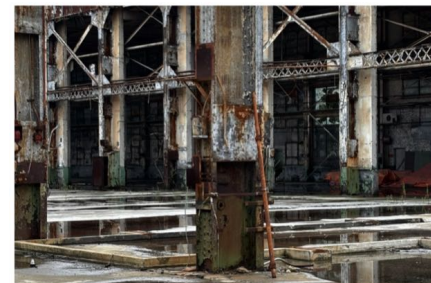
EXISTING STRUCTURE TYPICAL COLUMN BASE
