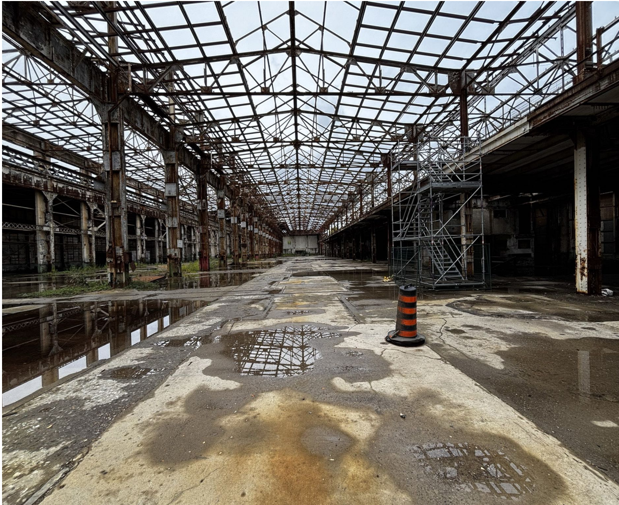
INTERIOR VIEW LOOKING WEST
